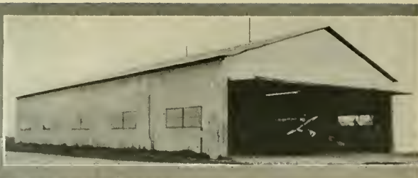
Steel and sheet metal hangar built in quantities from 1927 to 1929
